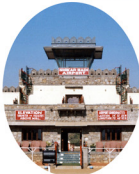
Air Traffic Control Tower
